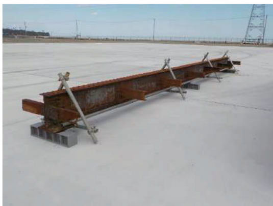
Fig.6 Viewing of steel rivet girder
