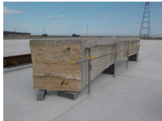
Fig.5 Viewing of setting RC-T girder
