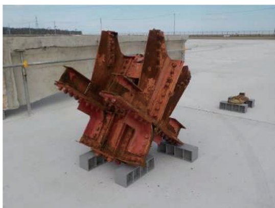
Fig.8 Viewing of panel point of truss bridge
