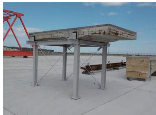
Fig.7 Viewing of RC-slab deck
