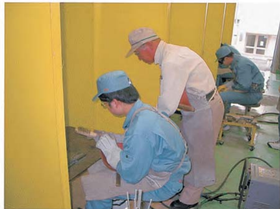
(b) Welding working
